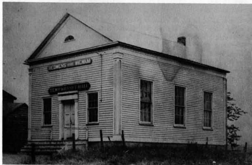
Illustration 2. For 136 years, travelers along the Western Turnpike (Route 20) passed Redmen's Hall. Built originally in 1809 as a Baptist church, it served at various times as St. Ambrose's Catholic Church, a temperance hall, the fraternal order of Redmen's Hall, and a community center. It burned in 1967.
