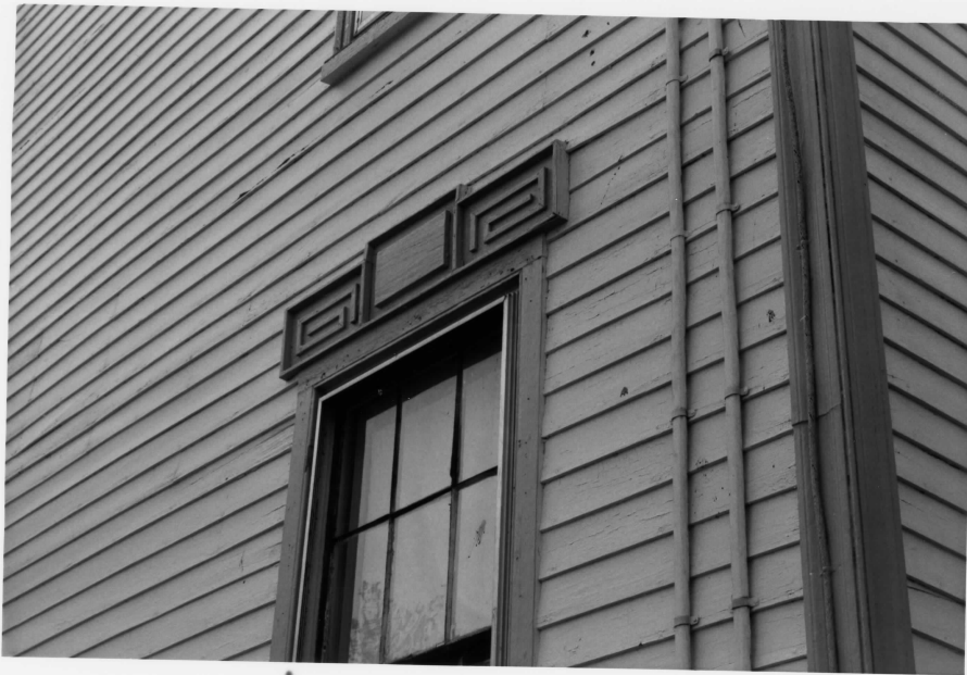
Detail of key design of window lintels
