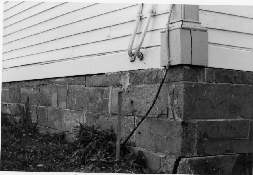
Detail of ashlar stone foundation
