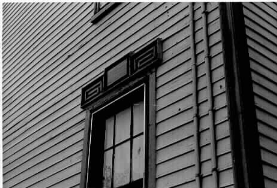
Detail of key design of window lintels
