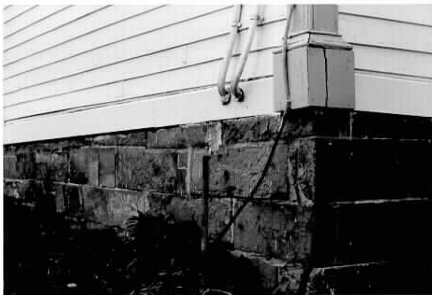
Detail of ashlar stone foundation
