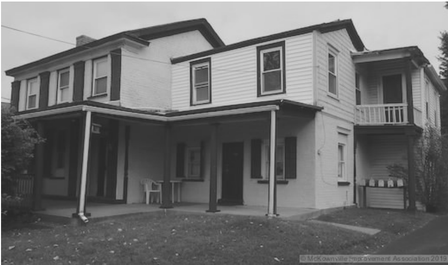
The Federal-style brick house at 1245 Western Avenue. Built by Eli Warford in 1850; occupied by Jacob Sager 1864-1870; sold to Charles Gimlick 1881. The oldest surviving house in McKownville.
